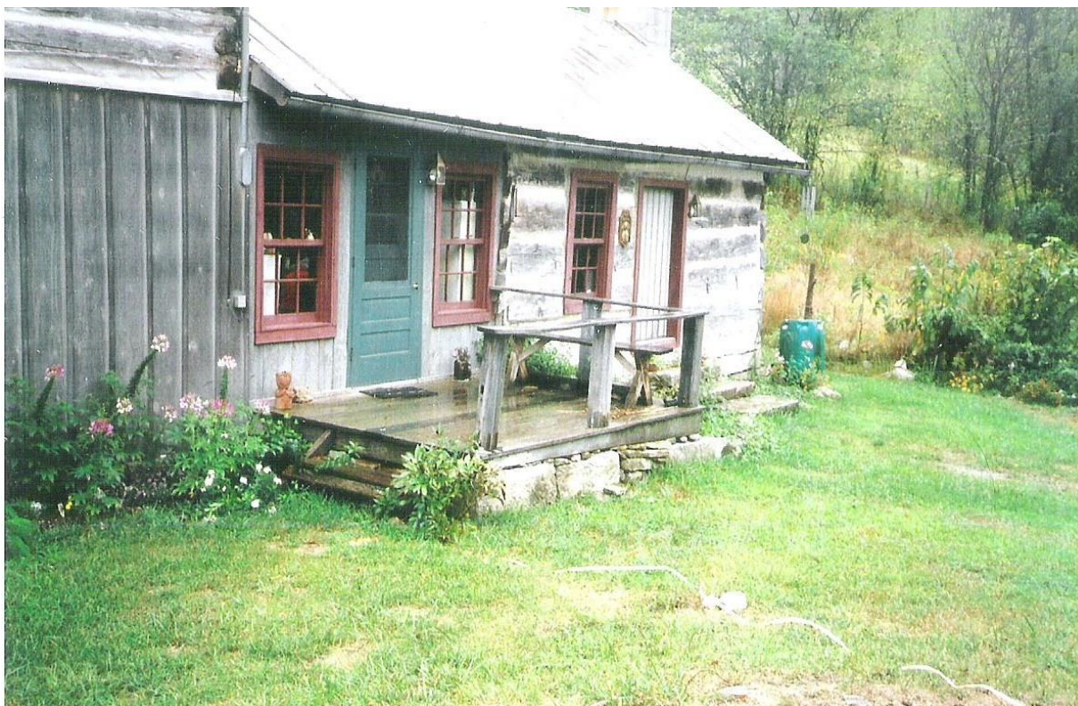
Front side of Kitchen, restored and remodeled, John Vaughan house; Mabel Harp Photo, 1997.
