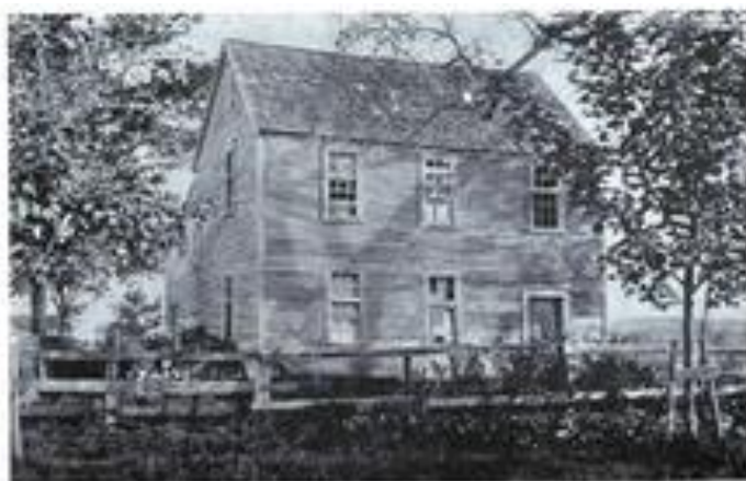
THE HOUSE BUILT BY WILLIAM SUTTON, NEW CASTLE, N.H.
